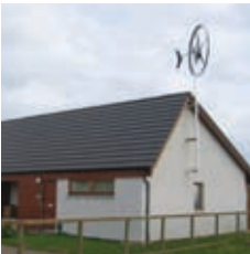
Building mounted SWIFT
