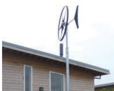
Stand alone steel pole
